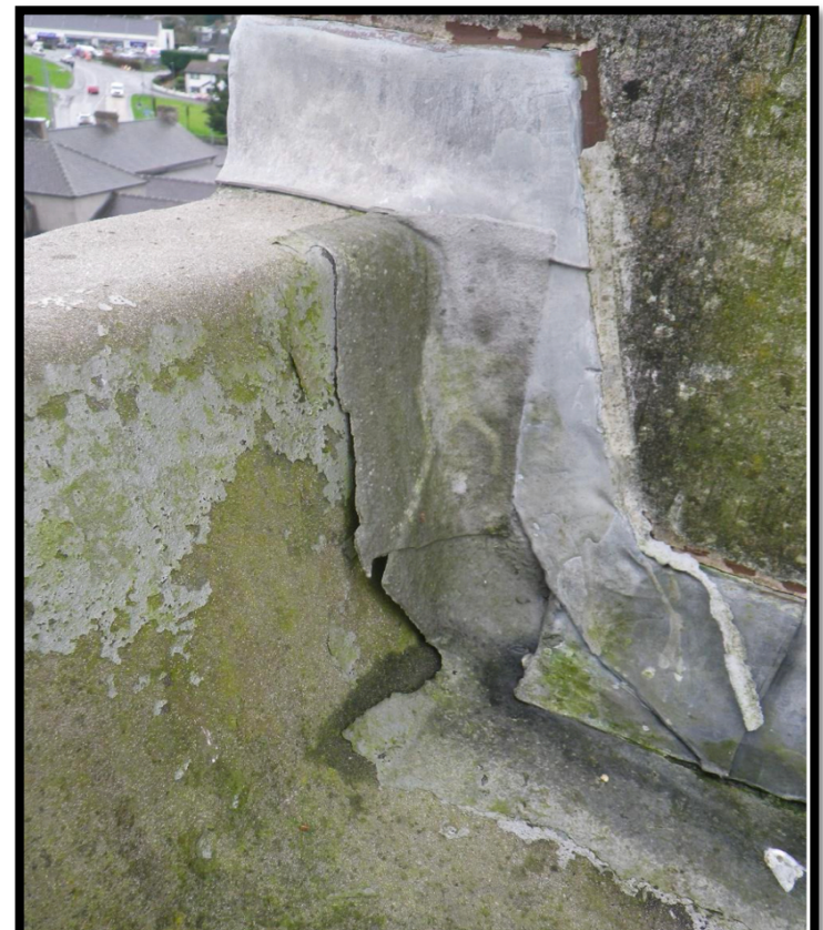
Poor past repairs to Tower roof
