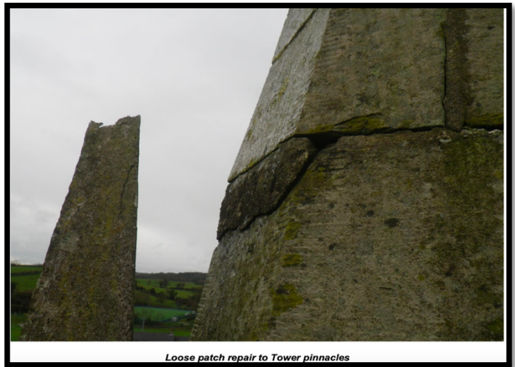
Loose patch repair to Tower pinnacles
